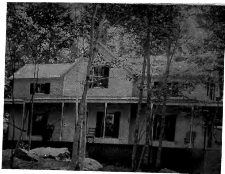
"The Birches" was built by William Munson and later owned by Nellie and Ed Hannum. It was torn down some years ago and the permanent home of Mr. and Mrs. Ralph Rudd III now stands on the lot.
